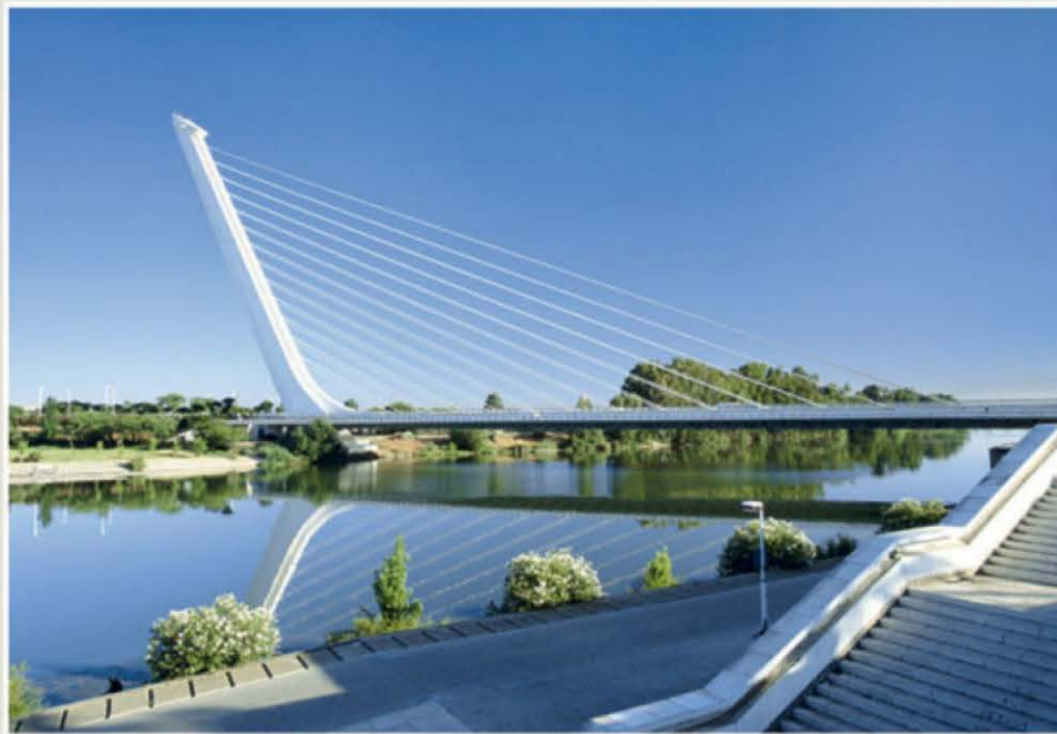
▲ Built for Expo 92, the Alamillo Bridge across the River Guadalquivir in Seville demonstrates how a striking new bridge can revitalise an old city. The bridge is supported by a pylon and cables which form the graceful shape of a harp. It has a span of 200 metres.
