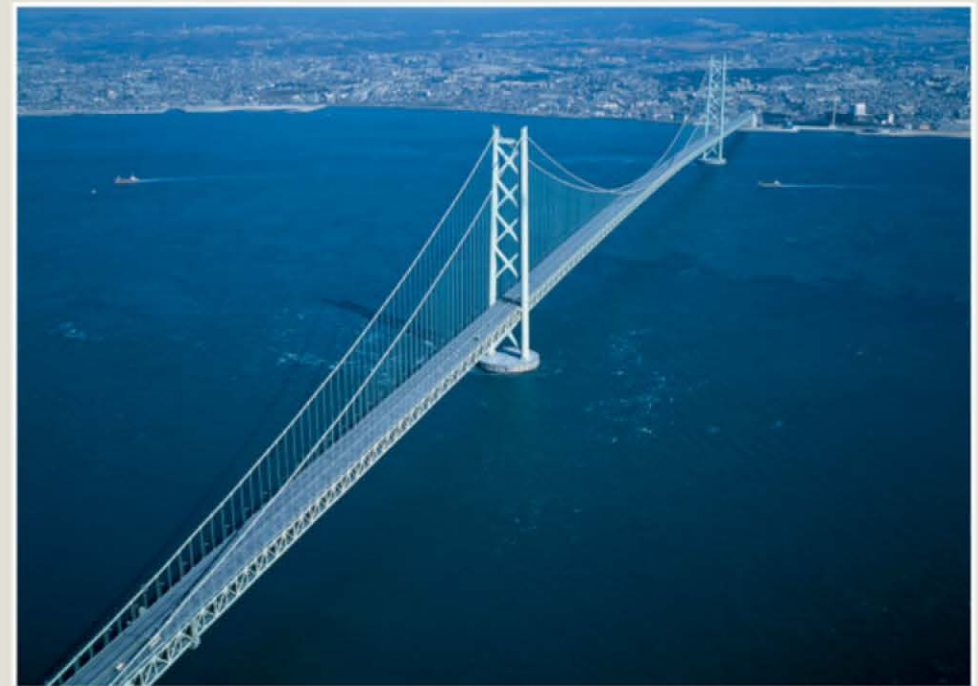
▲ The Akashi Kaikyo Bridge in Japan is the longest, tallest and costliest suspension bridge ever constructed. Connecting Kobe with Awaji-Shima Island, this bridge has been built to withstand hurricanes, tidal waves and earthquakes. In 1995, an earthquake added a metre to the bridge's length while it was still being built. It has a total length of 3,910 metres.
