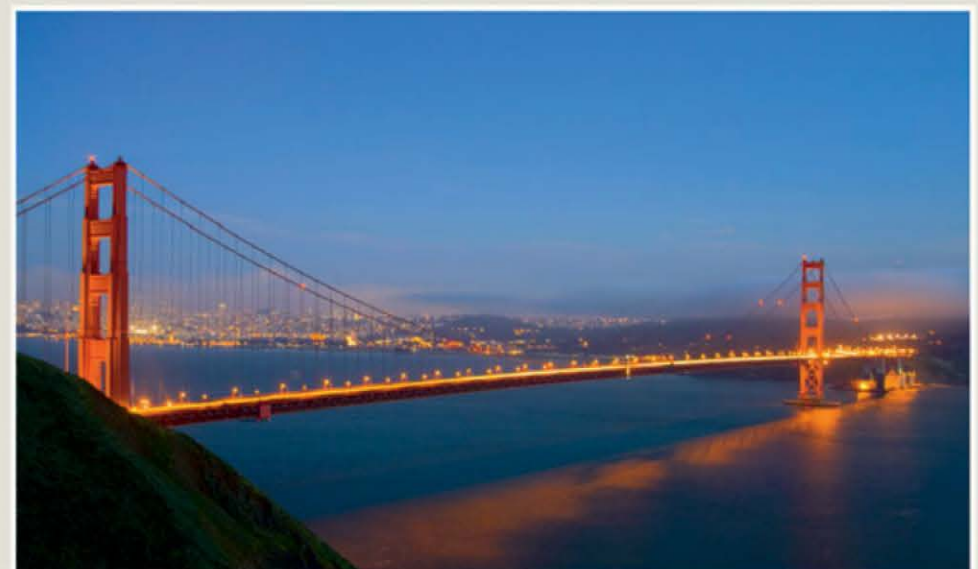
▲ The Golden Gate Bridge spans the mile-wide mouth of San Francisco Bay. The total length of the bridge is 2,739 metres. The bridge expands on hot days and contracts when it is cold. On hot days the heat lengthens the cable. As a result the bridge becomes 4.9 metres lower and 1.8 metres longer. The bridge was opened on 21 May 1937 with a 'pedestrians' day', during which 200,000 people walked across the bridge. On the morning of the following day it was opened to traffic.
