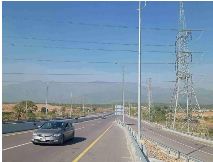
Figure 1- Electromagnetic radiation hazardous zone of road
